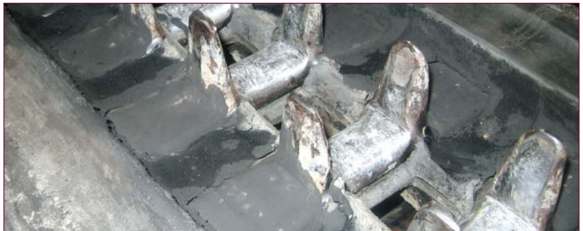
Below: This close-up view of the inside of the track shows the area that has been buffed away and cement has been applied to the steel cleats in the track.
